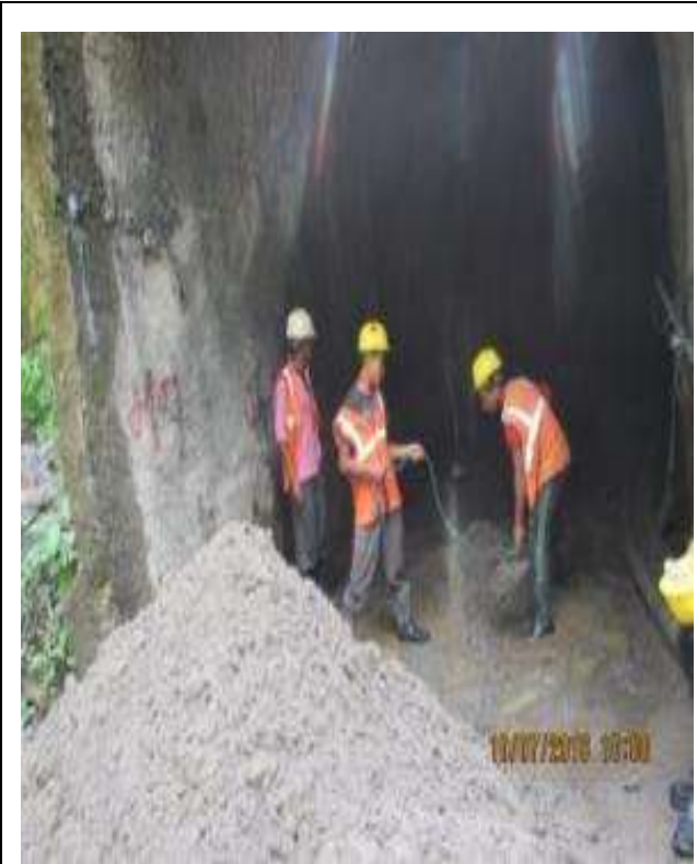
Dewatering diversion Tunnel
