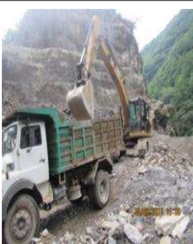
Mucking using a dump truck
