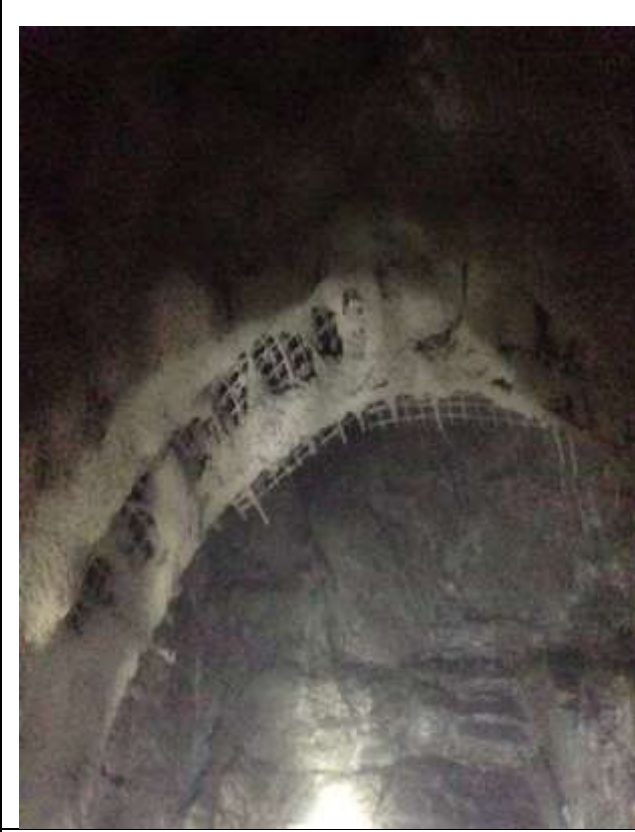
Installation of Primary Support
