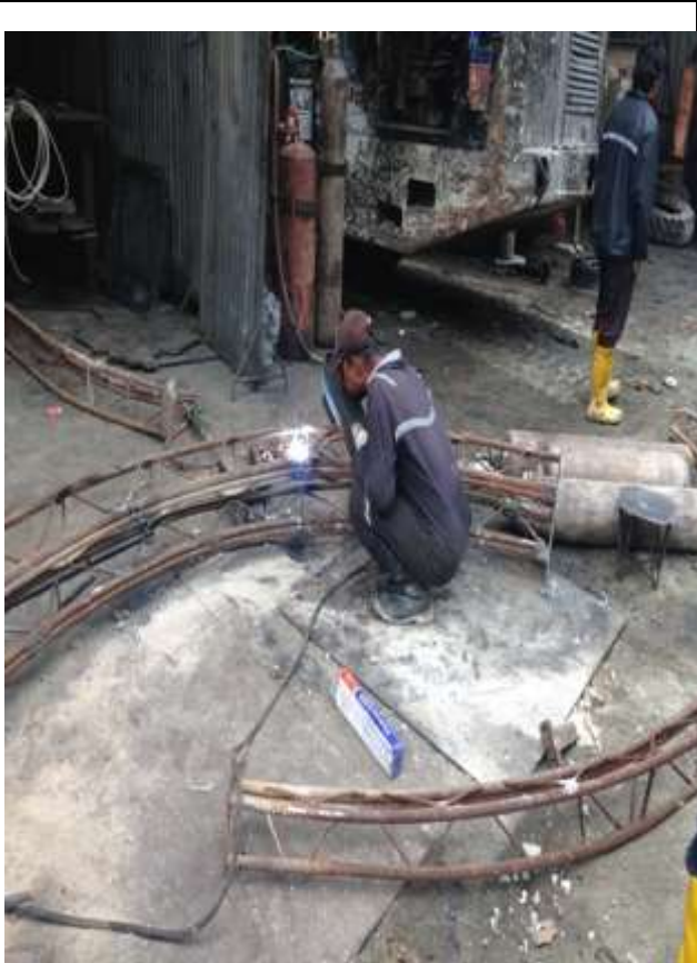
Fabrication of girder
