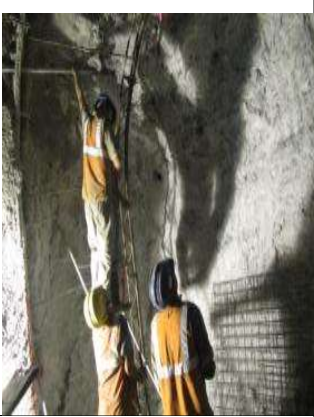
Installation of Primary Support
